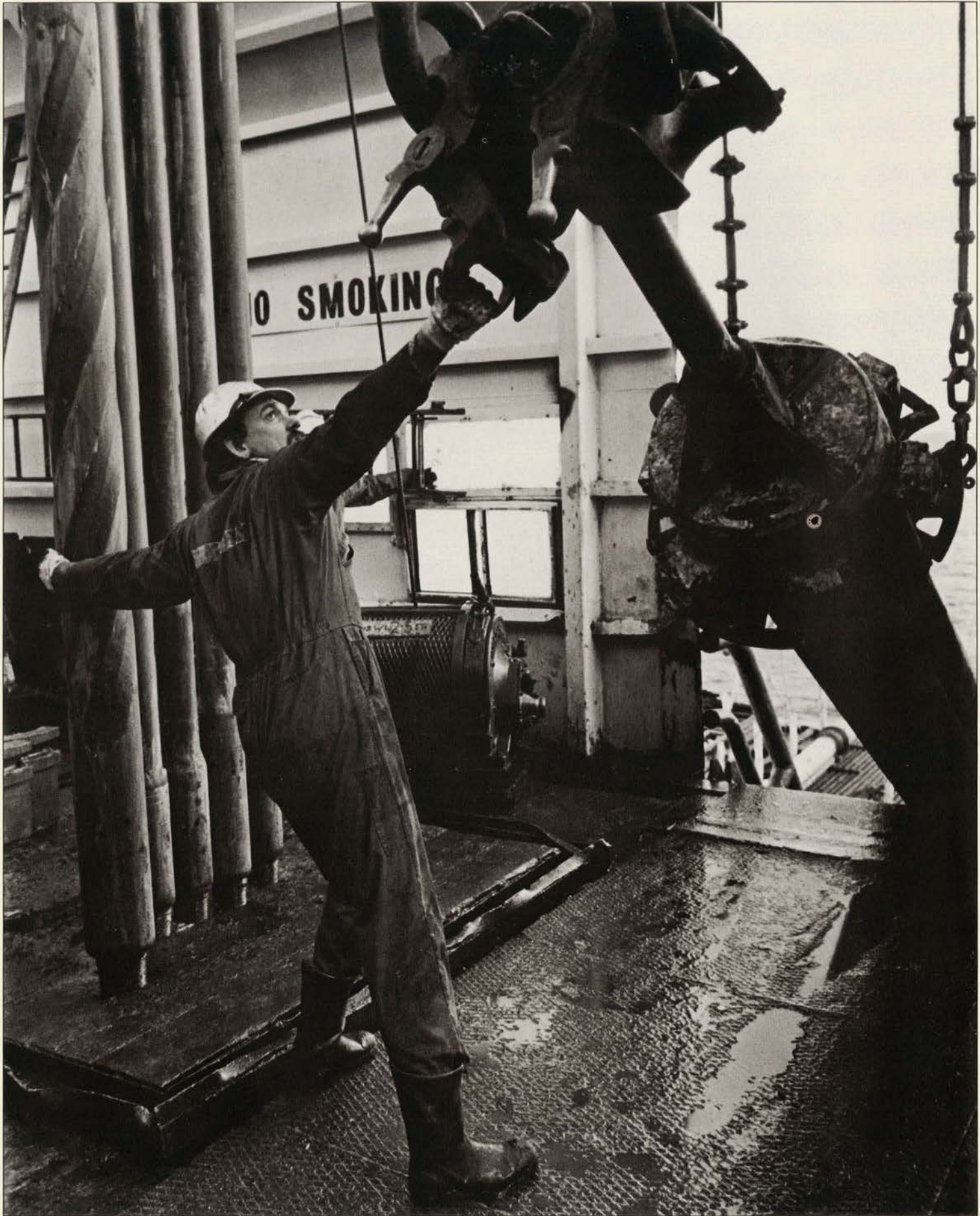
George Darby, assistant driller, unlatches drill pipe elevators to allow removal of a riser joint from the drill floor to a storage area.
