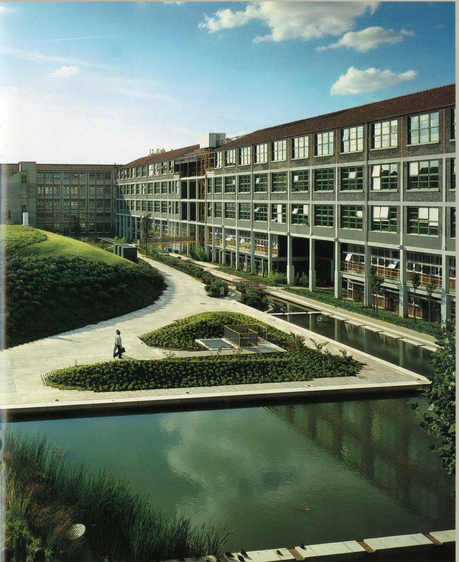
Montrouge/An administrative and manufacturing complex for eleven Schlumberger companies.
