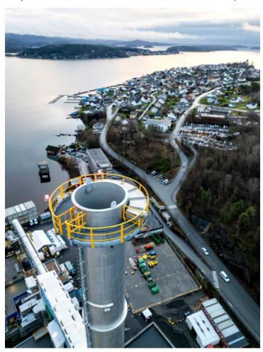
The carbon capture plant is designed to capture up to 400,000 metric tons of CO2 annually from the Heidelberg Materials cement facility in Brevik, Norway. (Photo: Business Wire)
